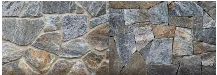
With vs. without mortar joint
